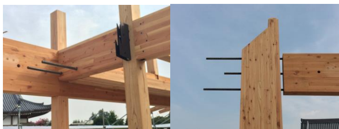
Figure15: T mode beam Joint
