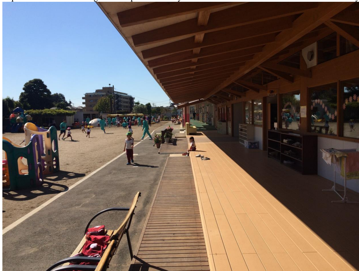
Figure2: Deep and long eaves sheltered children from the midday sun, yet free from structural obstacles.
