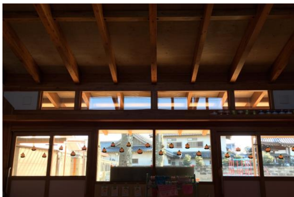
Figure13: Looking outside through the window
