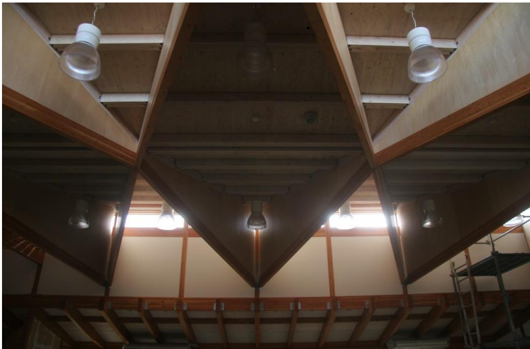
Figure 1: Looking up at the three dimensional frame of all-purpose room as a gymnasium and an assembly hall
