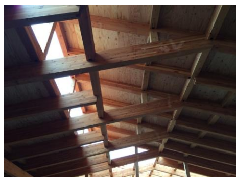
Figure4:Structure for high side lights
